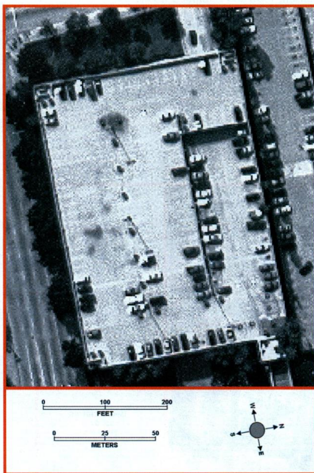
Figure 4 Light pole detection on top of parking garage.
